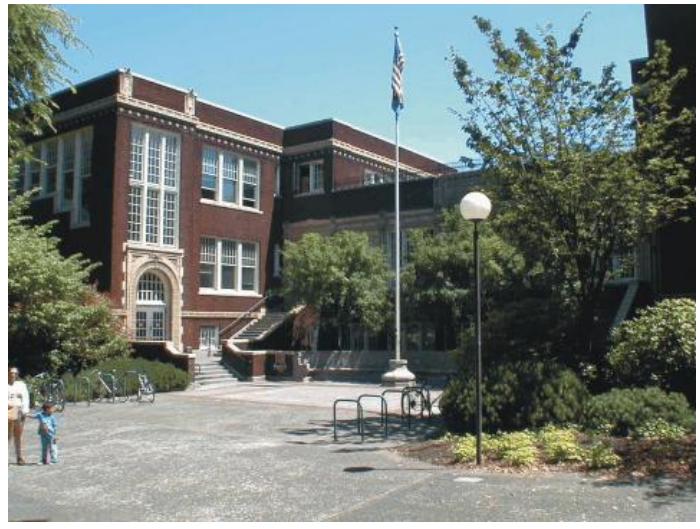
1914 SW Park Avenue, Portland, Oregon 97201
